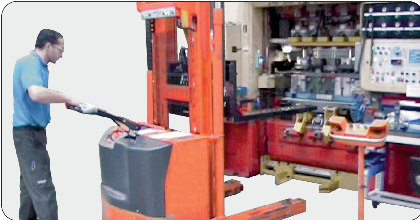
Tool-changeover on 120-tonne mechanical press fitted with a Rotobloc-PSP hydraulic tool-clamping system.
